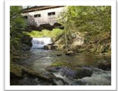
Bissell Bridge, Charlemont
